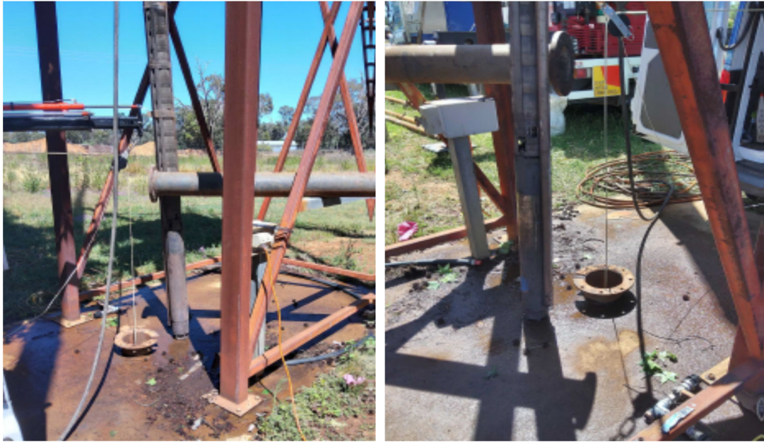
Condition of pumping equipment.
