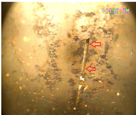
Slotted section at 190.70m and 191.80m.
